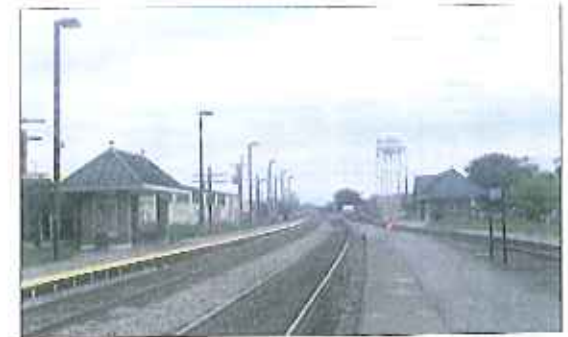
Station upgrades provide a new gateway for Elmwood Park.
